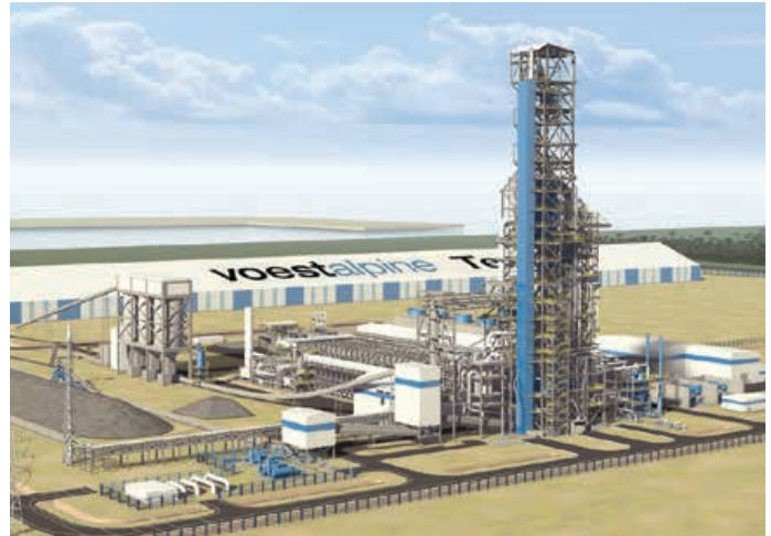
voestalpine Texas MIDREX® HBI Plant located near Corpus Christi, Texas, will be the world's largest HBI plant.
